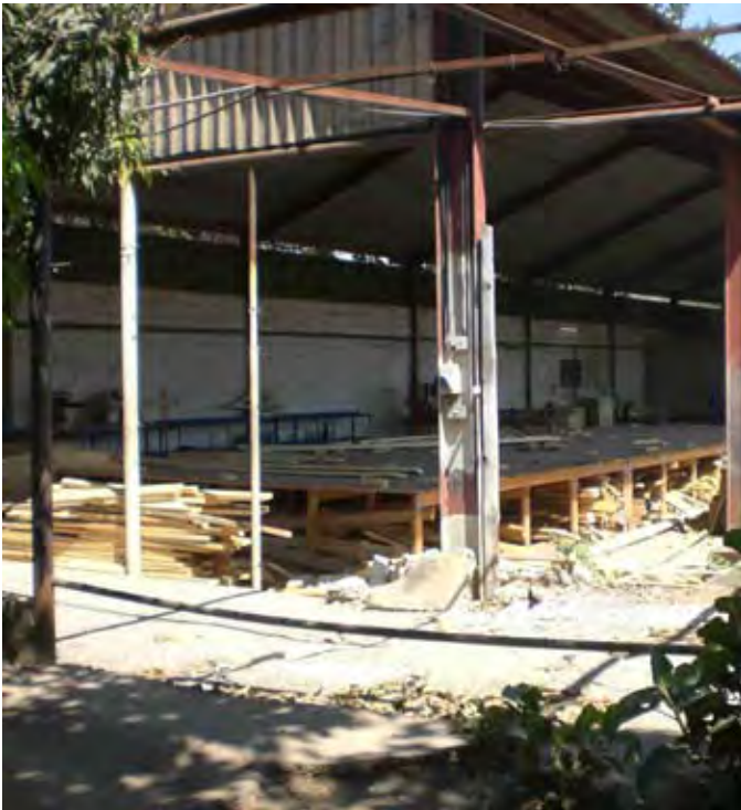
Kafakumba's dining center is under construction and will be built to "first world" standards.
